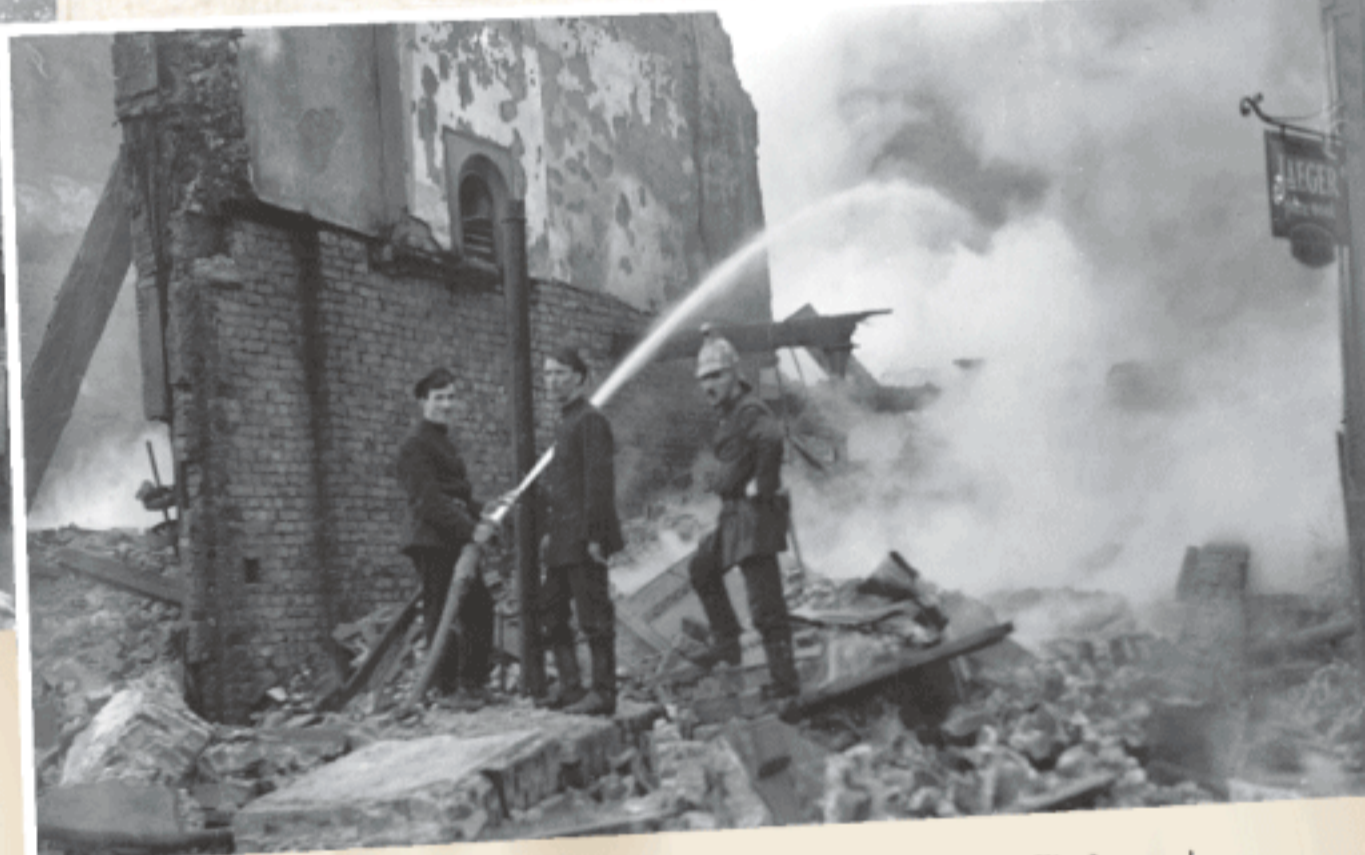
Firemen dealing with the aftermath of the previous night's fire at Cahill's drapers', 47 St Patrick's Street (on the corner with Princes Street) on Sunday, November 28, 1920. (Courtesy of Irish Examiner)
